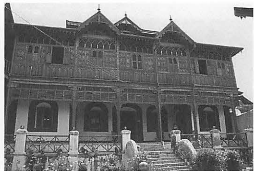
Fig. 5. The façade of the Rimbaud Culture Center
