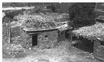
Fig 9. Hidmo roof where sheaf of straw is placed.
